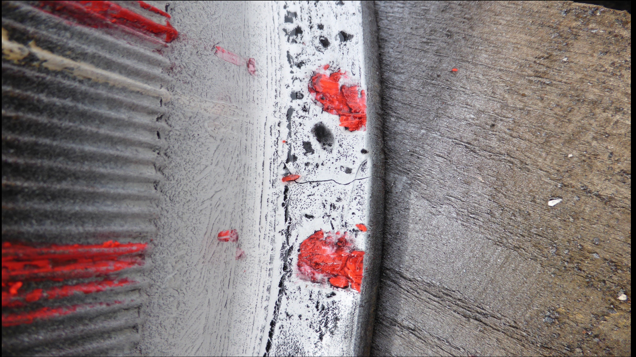
Figure 17: Crack in lip of Standard Back section
